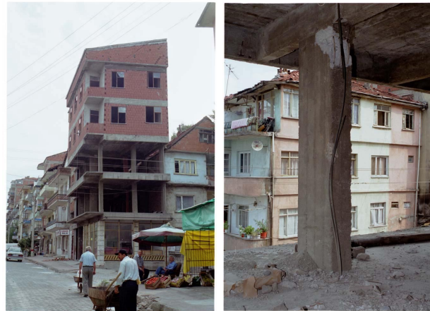
Photo 1. Whole view and damaged column of Building A (AIJ, 2001) 1) near Site E, which location is shown in Figure 1.
