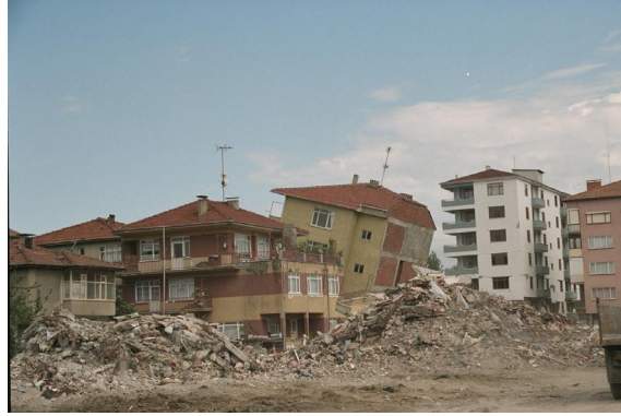
Photo 5.1. Damage to buildings in the northern area of Ataturk street.
