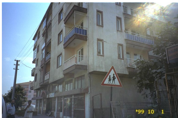
Photo 5.5. Heavily damaged building at which microtremor measurement was performed.
