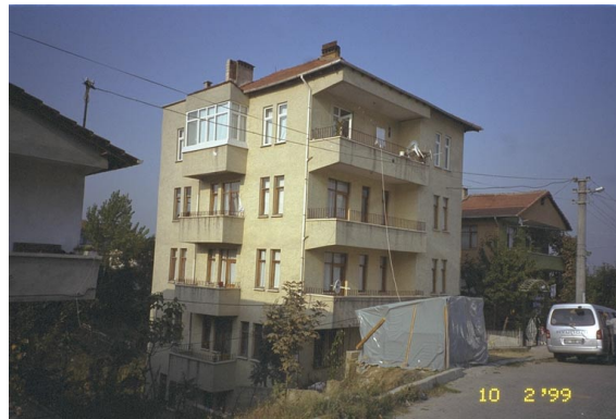
Photo 5.4. Non-damaged building that microtremor measurement was performed.
