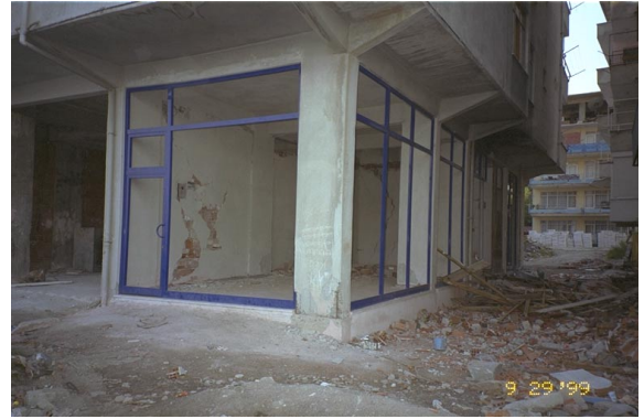
Photo 2.2.6. Rectangular cross-section column of commercial building, Golcuk.
