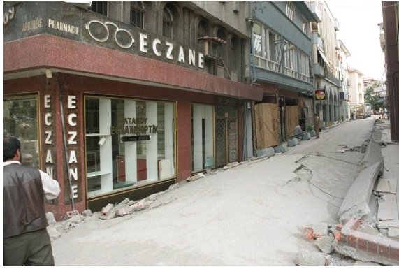
Photo 2.3.10. Up-heave of ground in Adapazari, Sep. 1999.
