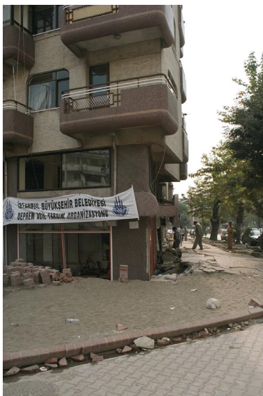
Photo 2.3.14. Settlement of Building C in Adapazari, Sep. 1999.
