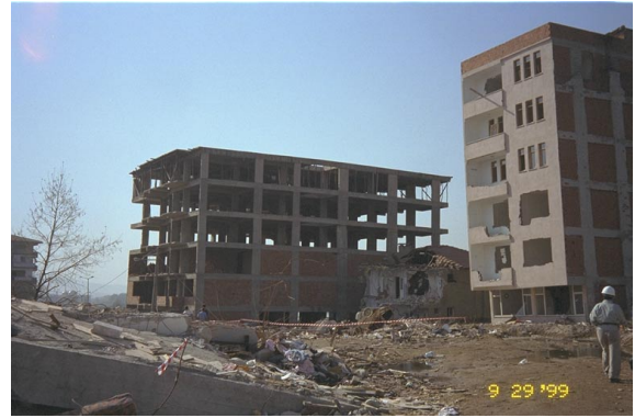
Photo 2.2.12. Submerged buildings and ground depression in Gölçük.
