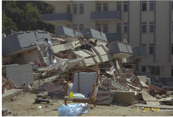
Photo 2.2.17. Pancake collapse of residence building, Yalova-Golcuk (Refer to color Photo 6).
