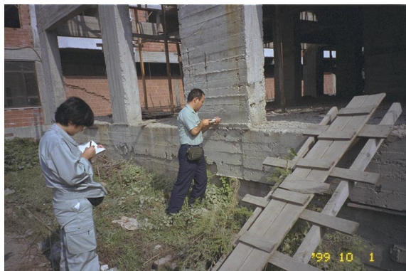
Photo 2.2.9. Schmitt hammer test at residence building, Sapanca.
