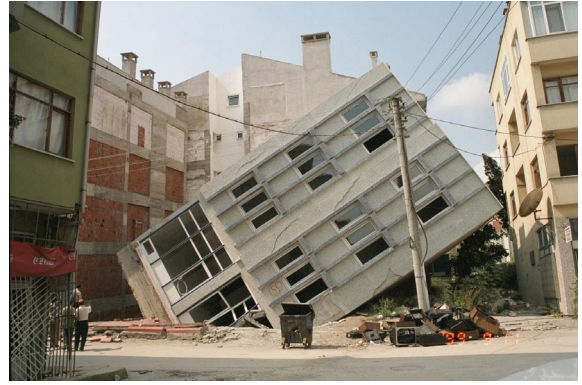
Photo 2.3.11. Inclination of Building A in Adapazari, Sep. 1999 (Refer to color Photo 12).
