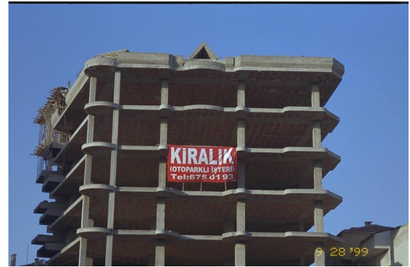
Photo 2.2.8. Flat infill slab in commercial building, Avcilar.
