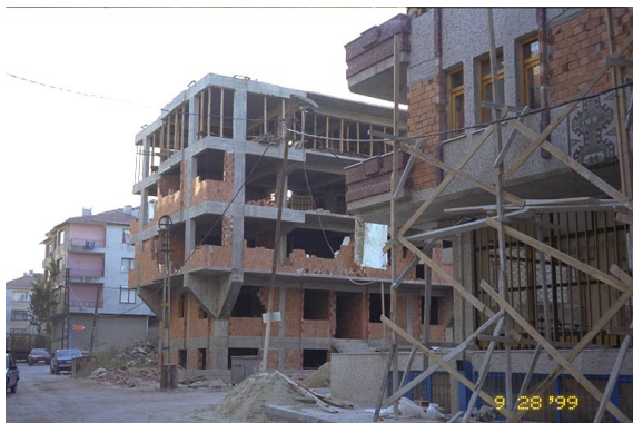
Photo 2.2.1. Mid-rise residence building under construction in Avcilar (Refer to color Photo 1).
