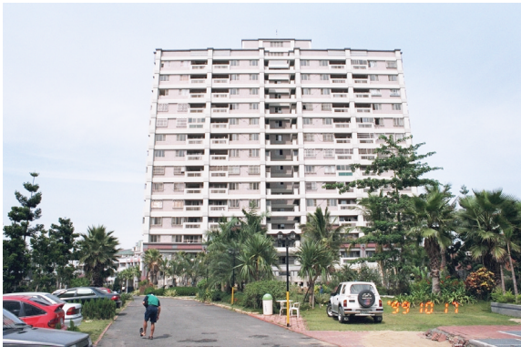
Photo 2.5.6. Subsided Building B in Nantou city.
