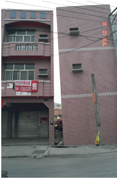
Photo 2.5.8. Inclination of Building D in Yuanlin district (Refer to color photo 12).
