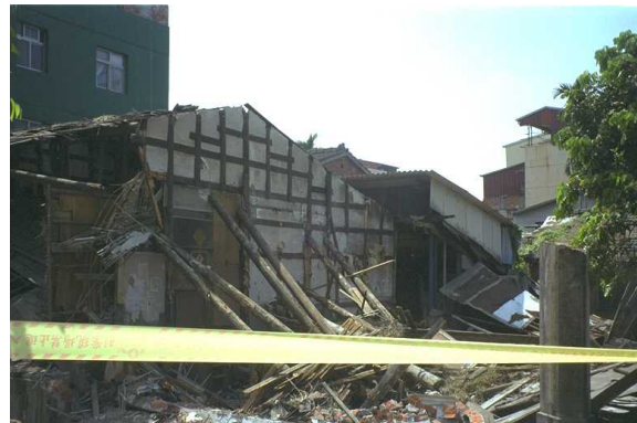
(b) Collapse of a building with earthen wall in Chi-Chi
