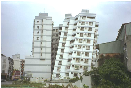
(a) Inclined apartment building (Refer to color photo 6)
