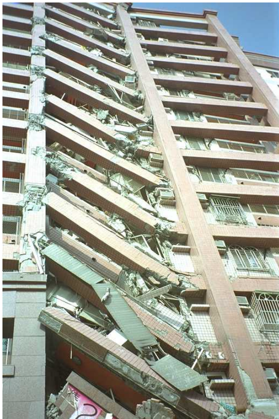
(a) Damage situation from the 2nd floor to the top floor
