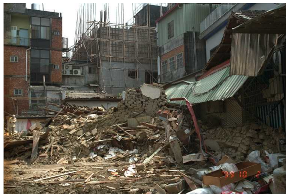
(c) Collapse of an earthen brick building in Tungshih
