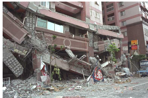
(b) Collapse part of first and second stories (Refer to color photo 5)
