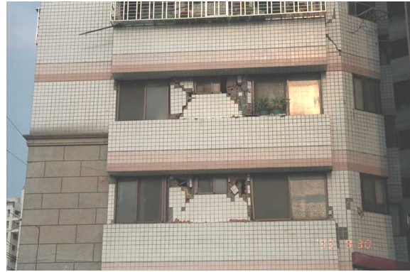
(b) Cracks on the wall
