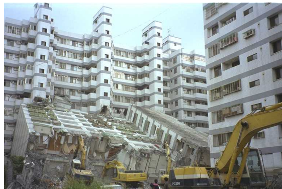
(b) Collapse of high-rise apartment building. One building out of four similar buildings was collapsed.
