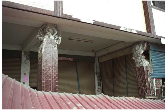
(b) Damaged pillar top of the first story
