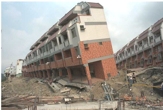
(a) Inclined building just on the fault rupture (Refer to color photo 9)
