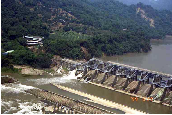
Photo 2.1.1 The Chelungpu fault running through the Shih-kang Dam site (Refer to color photo 15).
