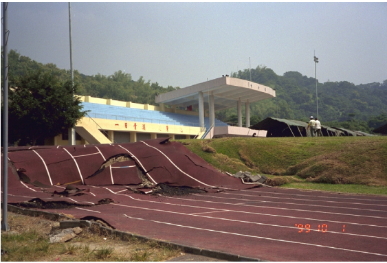
Photo 2.1.3 The Chelungpu fault running through the stadium in Wufeng (Refer to color photo 3).
