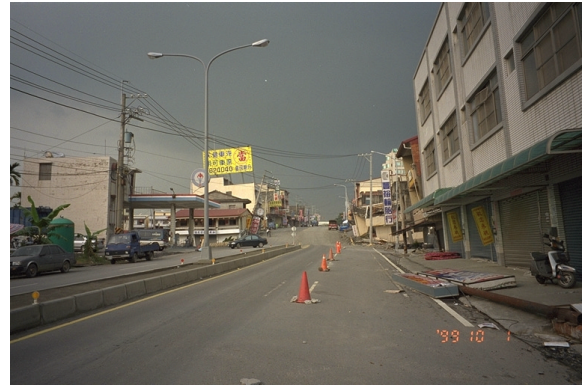
Photo 2.1.4 The Chelungpu fault running through the road in Chushan.
