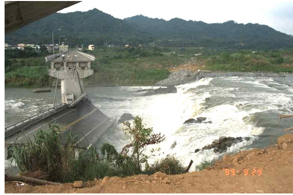
Photo 2.1.2 The Chelungpu fault running through the Pi-feng Bridge.
